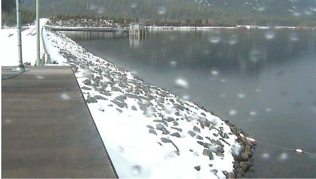
Sooke Lake Reservoir, from the top of the dam's spillway. February 2019
