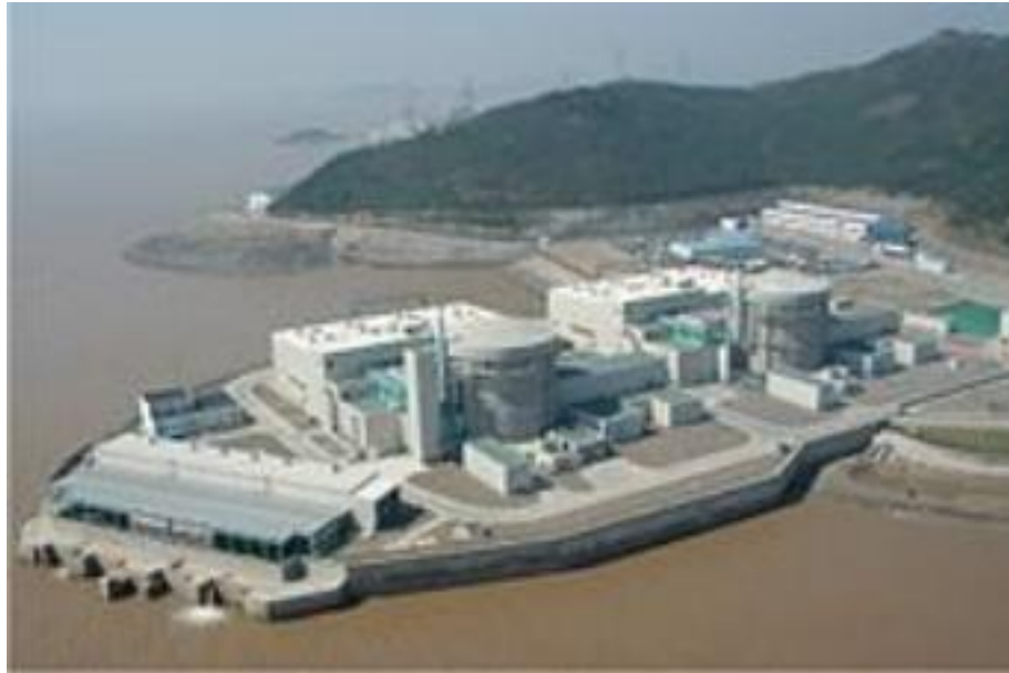
Qinshan Phase III Units 1 & 2
